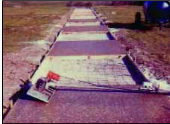
Finished sidewalk after it is washed.
